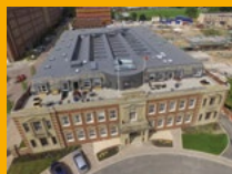
SINGLE PLY ROOFING
